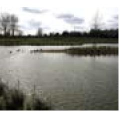
Sustainable urban drainage systems (SUDS) are widely used to reduce the impact of urban runoff on the aquatic environment. A permanent lake forms the basis for flood storage for the Quaggy Flood Alleviation Scheme in Kidbrooke, Greenwich
